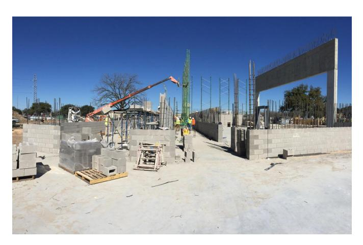
**BLOCK WALLS** – The block walls are being erected at the back of the stage, drama dressing rooms, costume storage and prop storage rooms.
