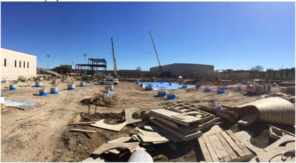
**PIERS** – The pier drilling work has been completed. Installation of mud slabs and moisture protection continues at the future Cafeteria, Library, Art Rooms and Special Needs Classrooms.
