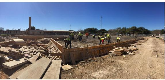
**FOUNDATION** – Mud slabs and moisture protection continue to be installed above. Concrete pours have been scheduled for the Career Technology Classrooms on February 12, 2016.
