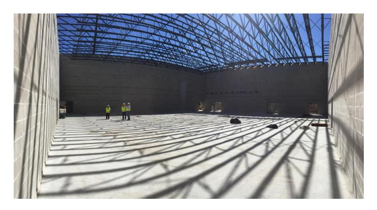
**STRUCTURAL** – Steel roof joists have been lifted and welded into place at the Auxiliary Gym. Installation of roof deck has started this week. Bleachers will be installed on only one side of the main basketball/volleyball courts.
