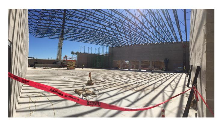
**STRUCTURAL** – Steel roof joists are being lifted and welded into place at the Main Gymnasium. Erection of the block walls continue on the east wall of the gymnasium. The south wall of the gymnasium has large window openings to the gymnasium lobby and concession area. Bleachers will be installed on both sides of the main basketball/volleyball playing courts.
